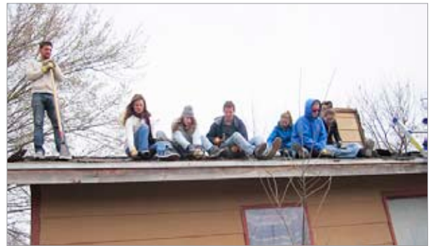
Below: Tearing shingles to repair the roof.
